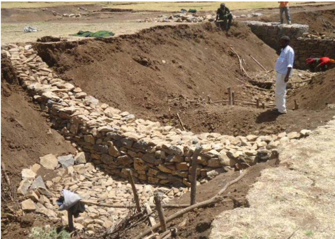
It is very important to extend the bottom and sides of the check dams about 15 cm into undisturbed soil, leave the center low for water to flow over, and construct an apron on the down-stream side of the dam to reduce the velocity of the overflow water and thereby reduce the hazard of water undercutting the dam. Building new check dams at higher elevations when sediments have filled the space behind the old check dams may gradually fill the gully.
